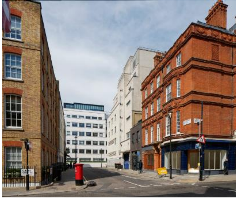
Existing view from Clifford Street, looking north-west:
